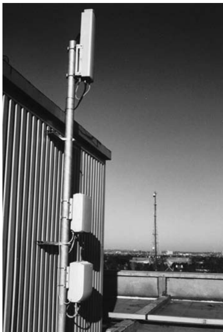
Figure 4.28 Roof-top mounted sector site consisting of antenna unit with integrated amplifiers, micro base station, and battery backup unit (Courtesy of Ericsson)
